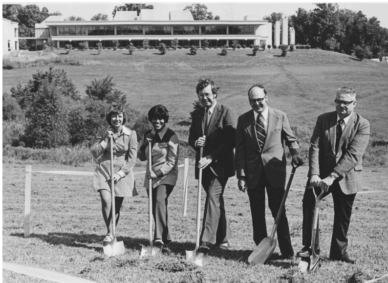
Edward Cochran, fourth from left, then Howard County executive, holds a shovel at the Howard Community College groundbreaking for the physical education complex. (Columbia MD Archives)
